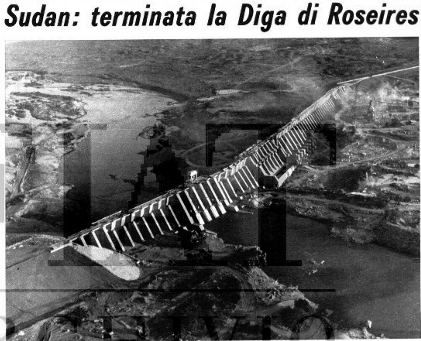
1,111,800 cu yd in volume — took four years to complete. Forming a lake of 5,886,000 cu yd, it was built to harness the floods of the Blue Nile and to provide irrigation water. The project was designed to permit the supply of water to the huge power station, moved by 7 turbo-alternator units of 25,000 kW each, located at the foot of the barrage. The wall, in concrete, extends on both sides into 8½-mile-long berms of earth with a volume of 5,362,800 cu yd.
