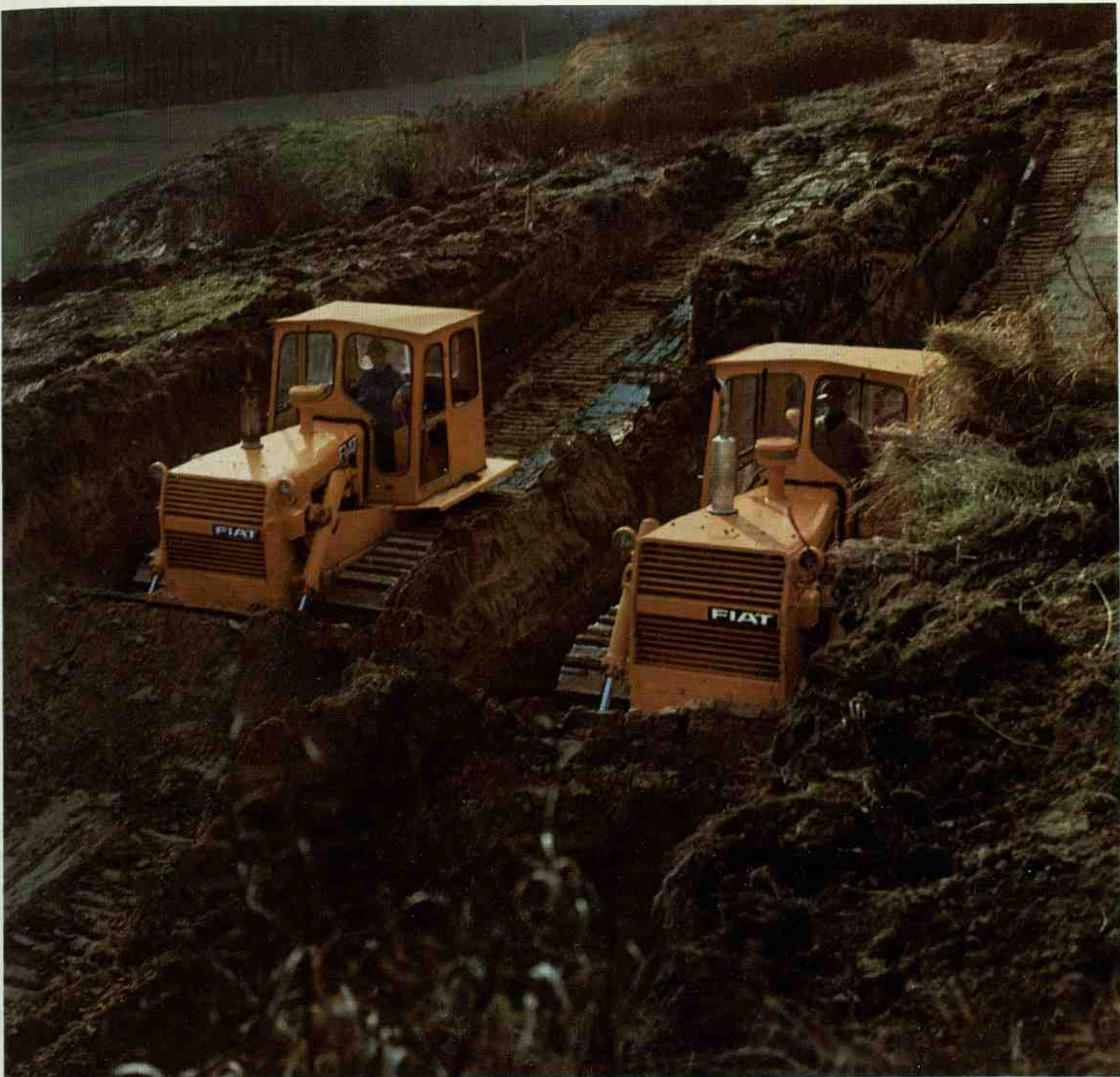
Fiat earthmoving machinery engaged in land clearing work near Fribourg, West Germany.
