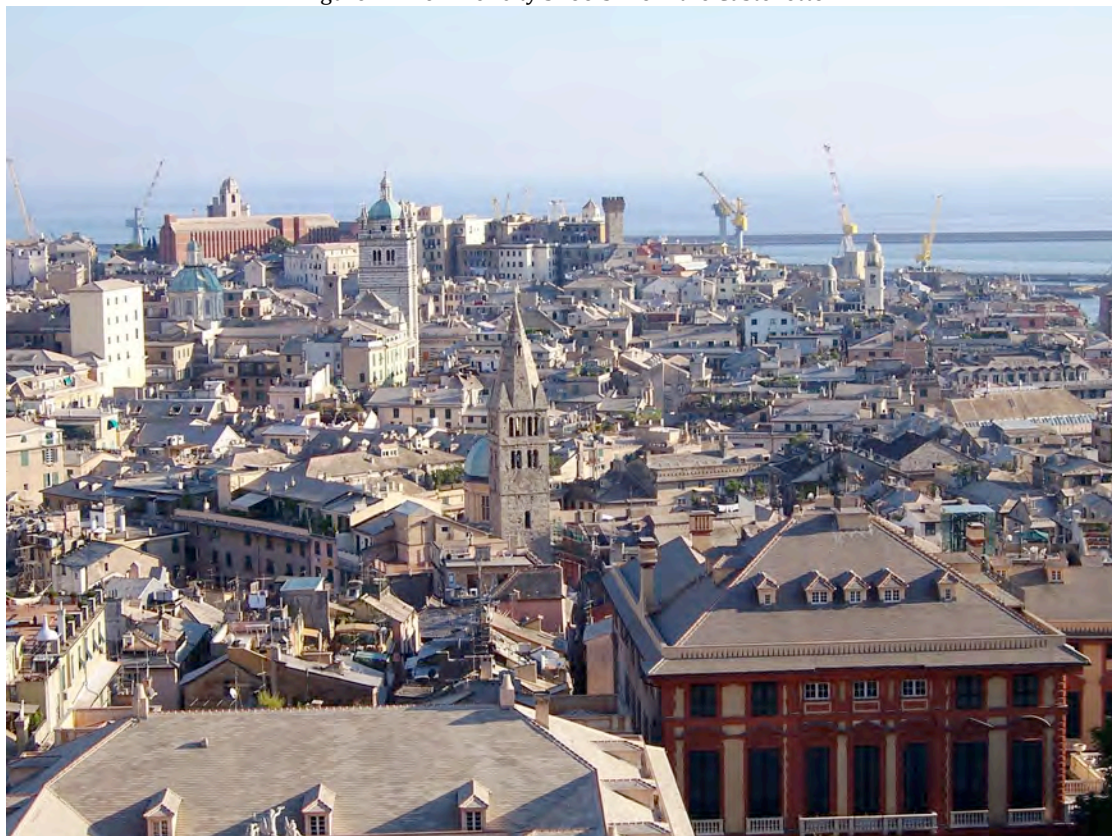
Figure 2. The inner city's roofs from the Castelletto
